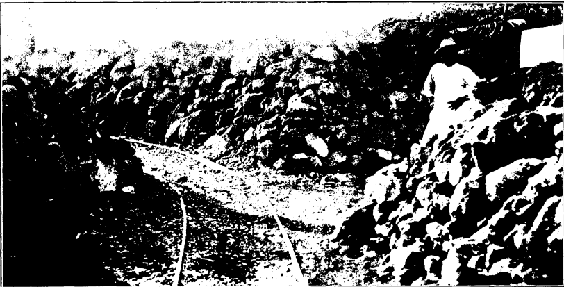
Fig. 3. Asphalt ready for shipment.
